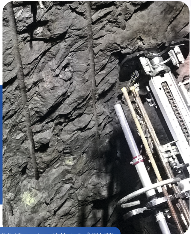
Self-drilling anchor with MasterRoc® RBA 380
